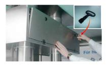
**1** The extract air box is opened with an allen key. Then lower the lid carefully.
