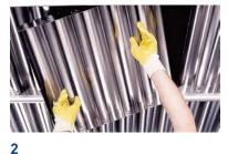
Carefully remove the cassettes from the C-profiles. Only hold the cassettes by the side plates or the small registers.
