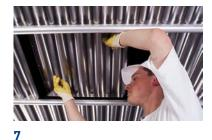
Insert the clean cassettes carefully into the C-profiles, linking one to another, and push them away one after the other (max. 10 cassettes) until the row is complete again.
